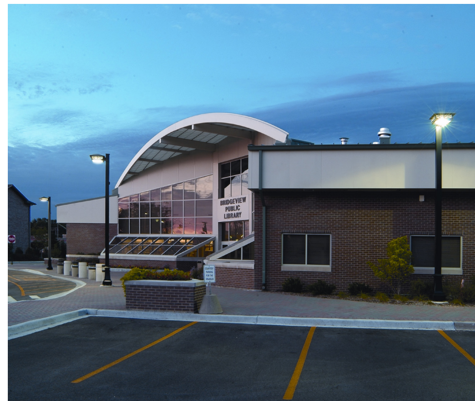
FIGURE 1.06 EXTERIOR LIGHTING EXAMPLES
