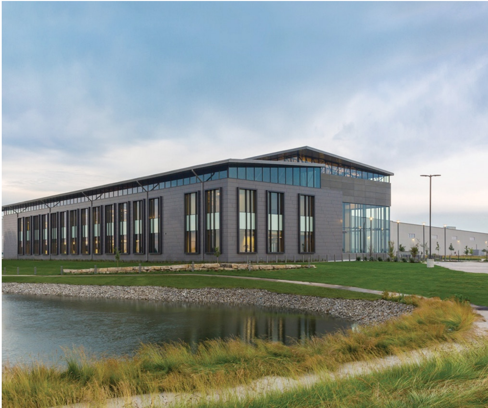
FIGURE 1.07 QUIK TRIP DISTRIBUTION CENTER, BELTON, MISSOURI
