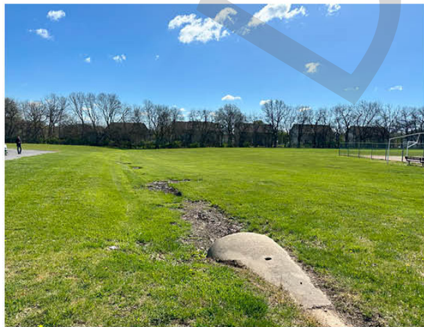
Erosion control measures need off of parking lot.
