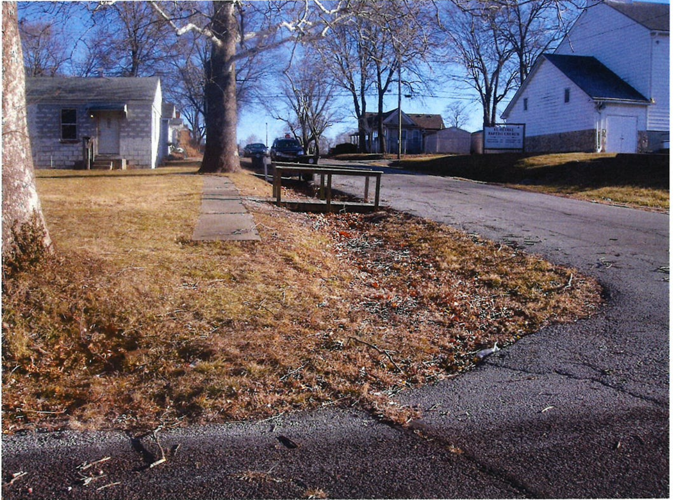
Photo 35- Image open storm water drainage ditch. It appears that some type of remedial access method has occurred with the presence of “pedestrian walkway”. Note lack of pedestrian sidewalk continuation and deteriorated nature of sidewalk.
