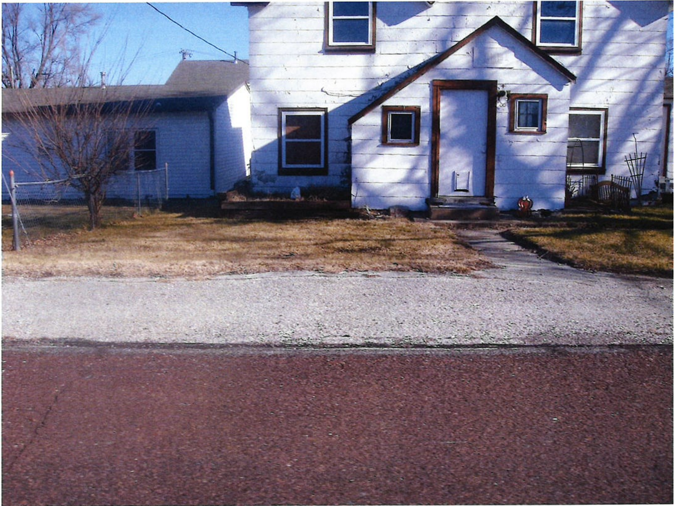
Photo 50 - Deteriorated single-family residence. Note broken and missing exterior shingling materials. Siding appears to be suspect asbestos-containing materials typical of this vintage construction.
