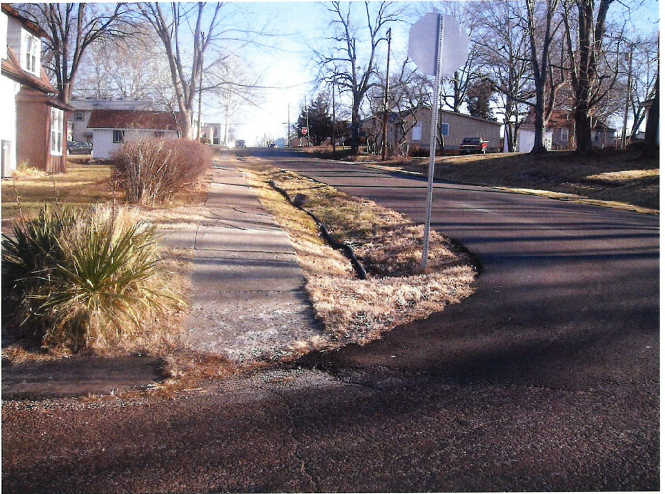
Photo 34 - Image open storm water drainage ditch. It appears that some type of remedial drainage has occurred with the presence of drainpipe along the surface. Note lack of pedestrian sidewalk continuation and deteriorated nature of sidewalk. Also note lack of truncated pedestrian strip at sidewalk crossing
