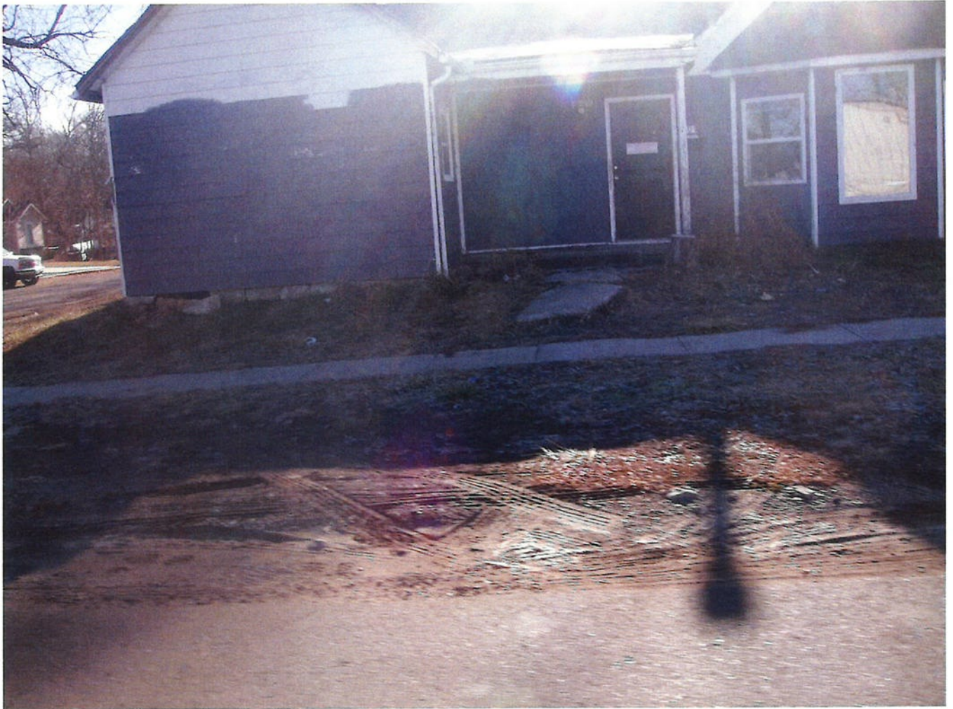
Photo 47 - Deteriorated single-family residence. Condition is an indication of lack of regular property maintenance. This condition may lead to an economic and social liability and may be conducive to the ability to pay reasonable taxes.
