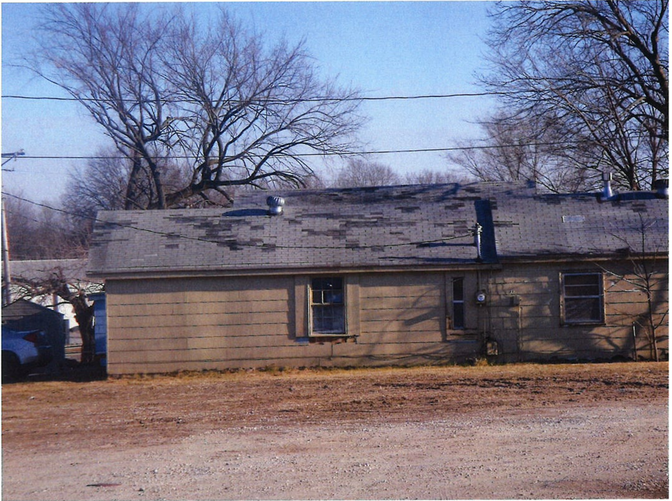
Photo 49 - Deteriorated roofing system, single-family residence. Also note broken and missing exterior shingling materials. Both are an indication of lack of regular property maintenance. This condition may lead to an economic and social liability and may be conducive to the ability to pay reasonable taxes.
