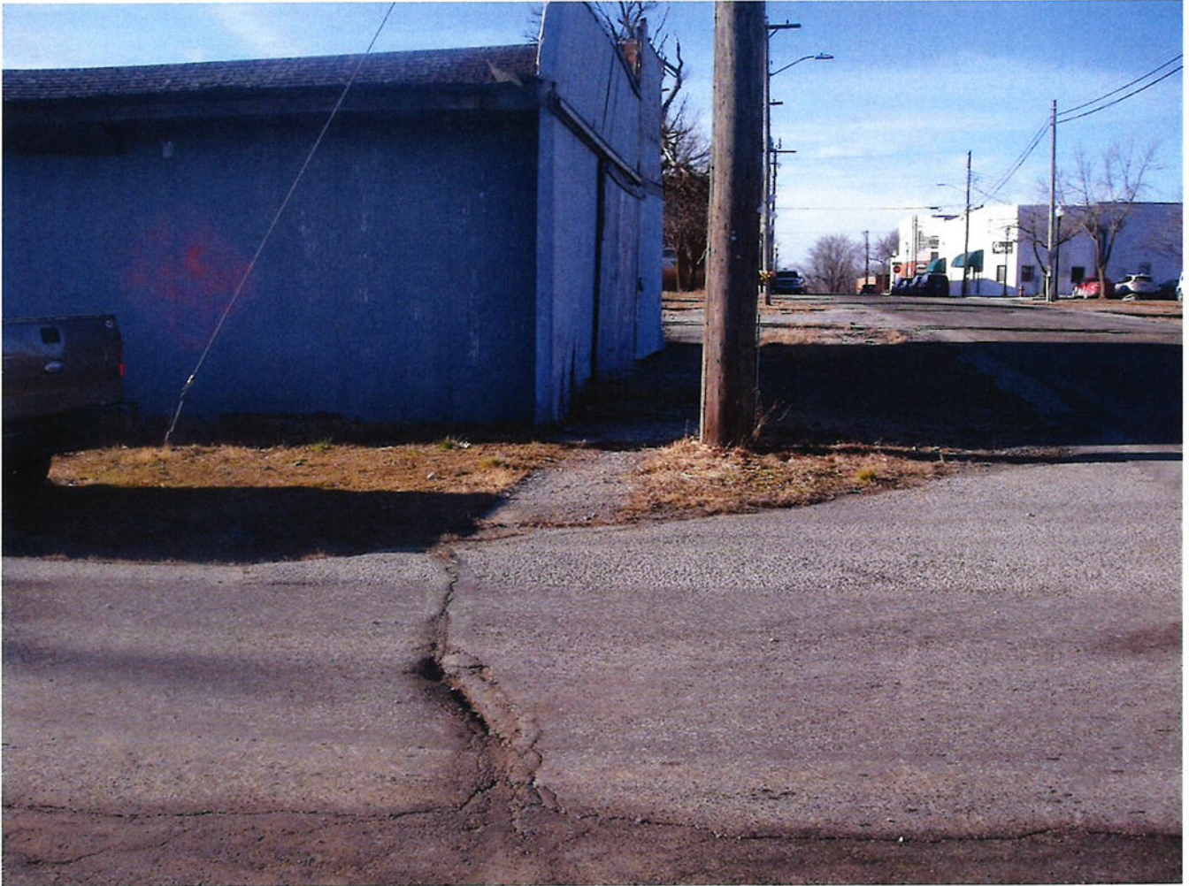
Photo 29 – View of inadequate pedestrian sidewalk infrastructure.
