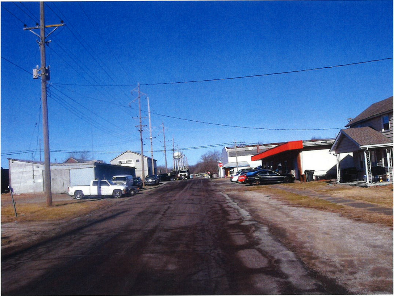
Photo 30 - Deteriorated/damaged sidewalk. It appears that vehicle repair activities are occurring over the sidewalk location and public right of way.
