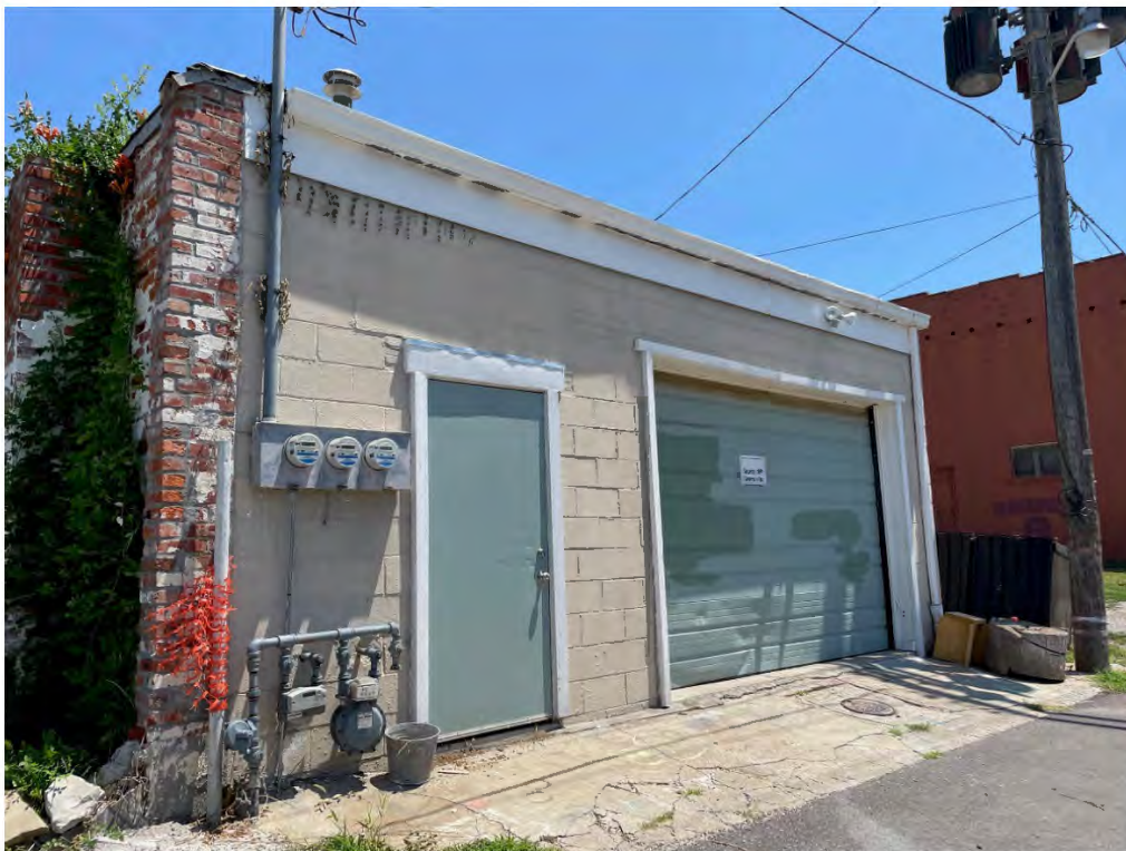
Rear/alley wall photo (repainting)
