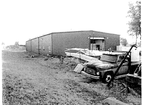
Photo #4 Maintenance building facing northeast
