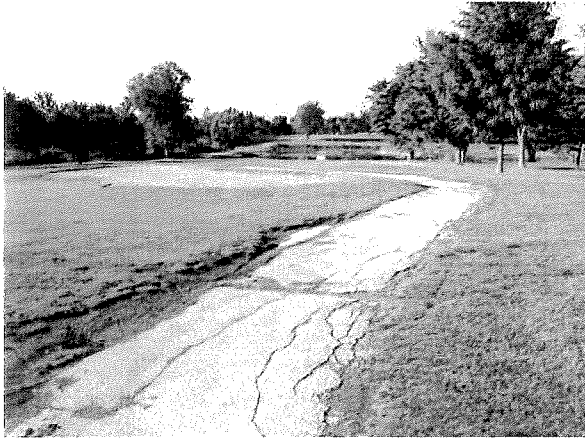
Photo #13 Facing south from the northeast corner of the site
