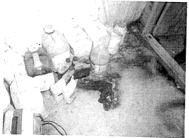
Photo #68 Inside the pesticide room, minor staining and no secondary containment
