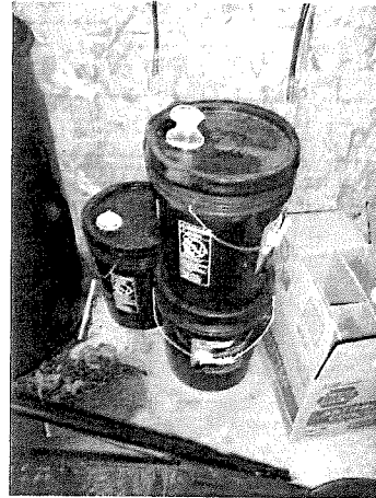
Photo #80 5-gallon containers of hydraulic fluid, and staining near the 55-gallon drum of new oil
