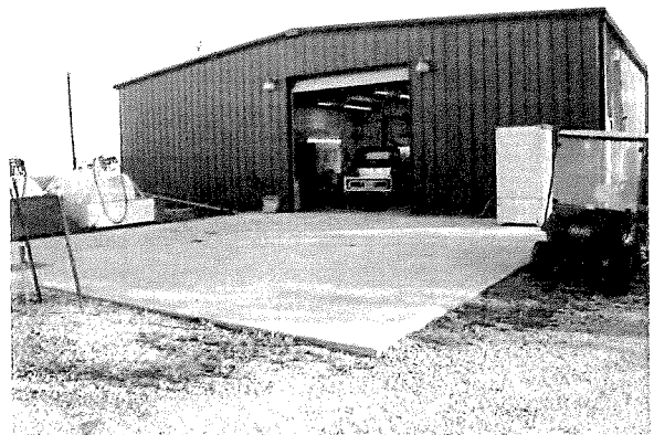
Photo #6 Maintenance building facing northwest
