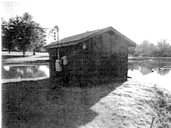
Photo #9 Pump house on the east-central portion of the site
