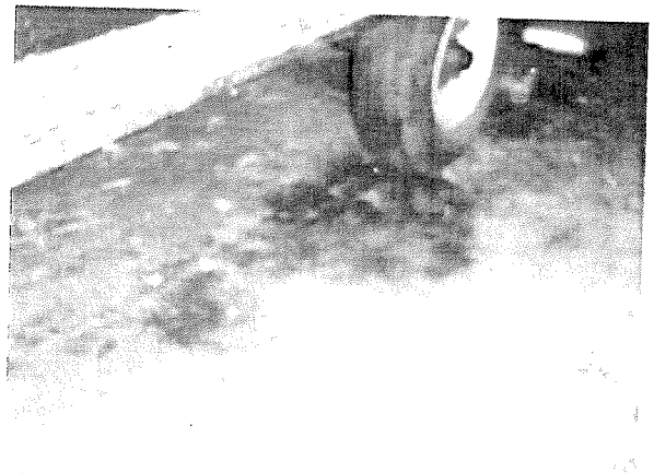
Photo #54 Staining on the soil in the south portion of the shed
