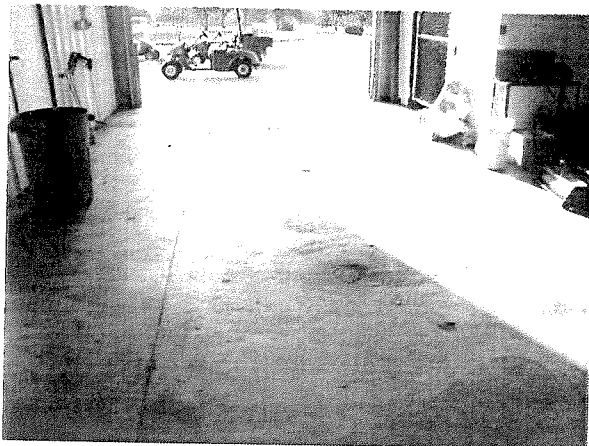
Photo #73 East bay door in the south portion of the building and floor drain
