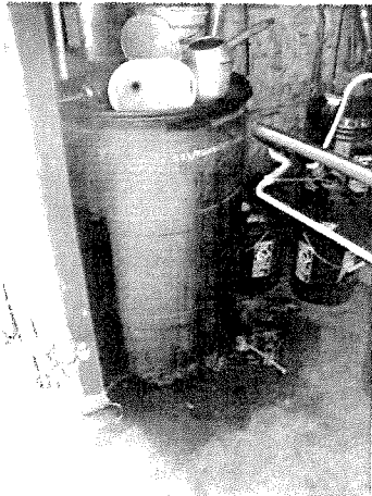
Photo #79 55-gallon drum of new oil with staining on the concrete
