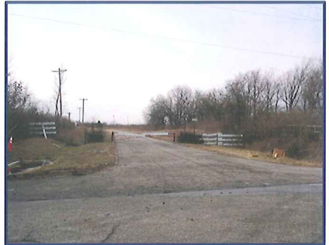
Looking south along Bales Road
