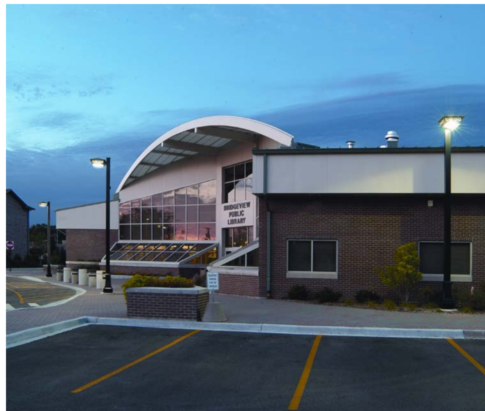
FIGURE 1.06 EXTERIOR LIGHTING EXAMPLES
